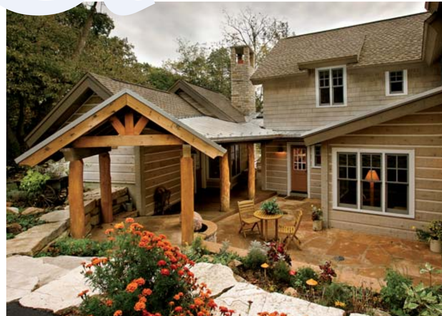
The hand-hewn cedar (above) was treated with a bleaching stain that will turn the exterior to a maintenance-free soft, silver gray over time. Hand-chinking gives the home a true old-time appearance.
