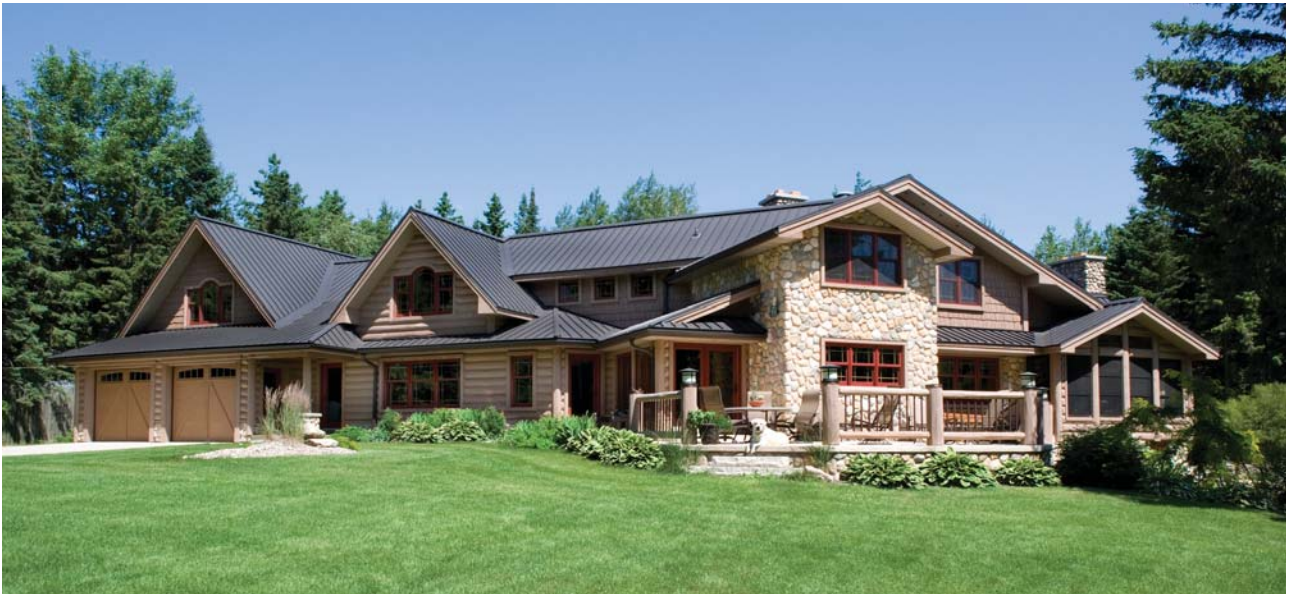
Above: The Wisconsin Log Homes Boulder Ridge plan was customized by the homeowners to incorporate architectural stone, shingles, and logs.
