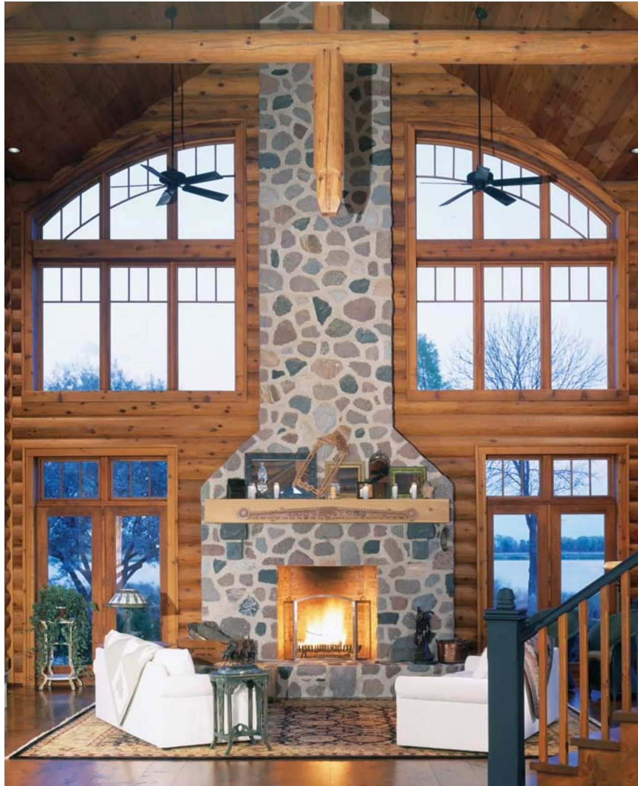
Above: A 30-foot fireplace with a timber mantel and symmetrical window display can be seen when guests enter the foyer, and the view continues to the waterfront view beyond. To balance the volume of the great room, 12-inch half-logs were used on the walls. A cedar-lined ceiling is accented with log trusses and extended king posts.
