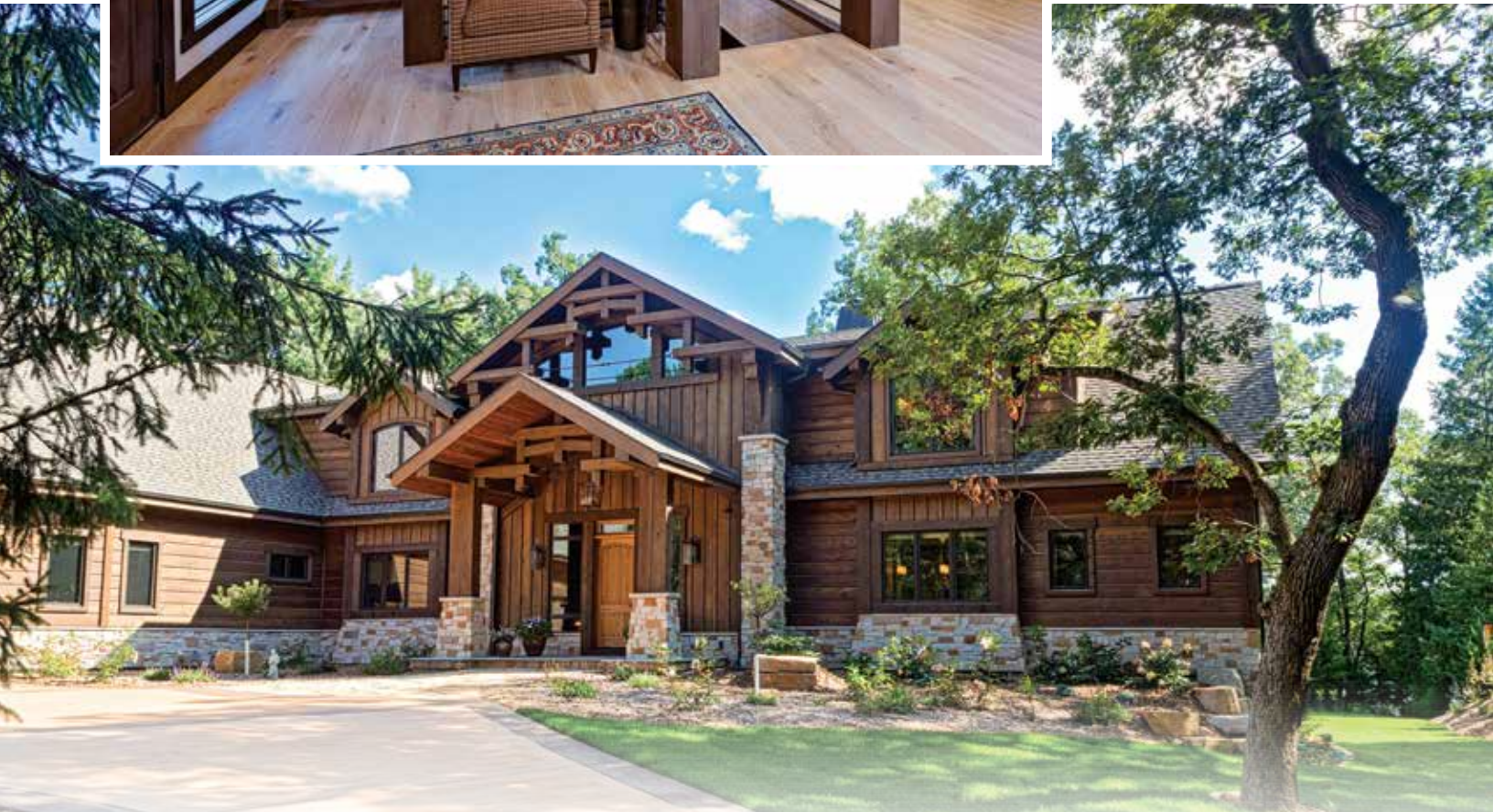
BELOW: The scope of the home required that it be treated as a commercial-grade structure in many ways. Areas of the house are framed out with 2-by-8 glue-lam construction to accommodate its size.
